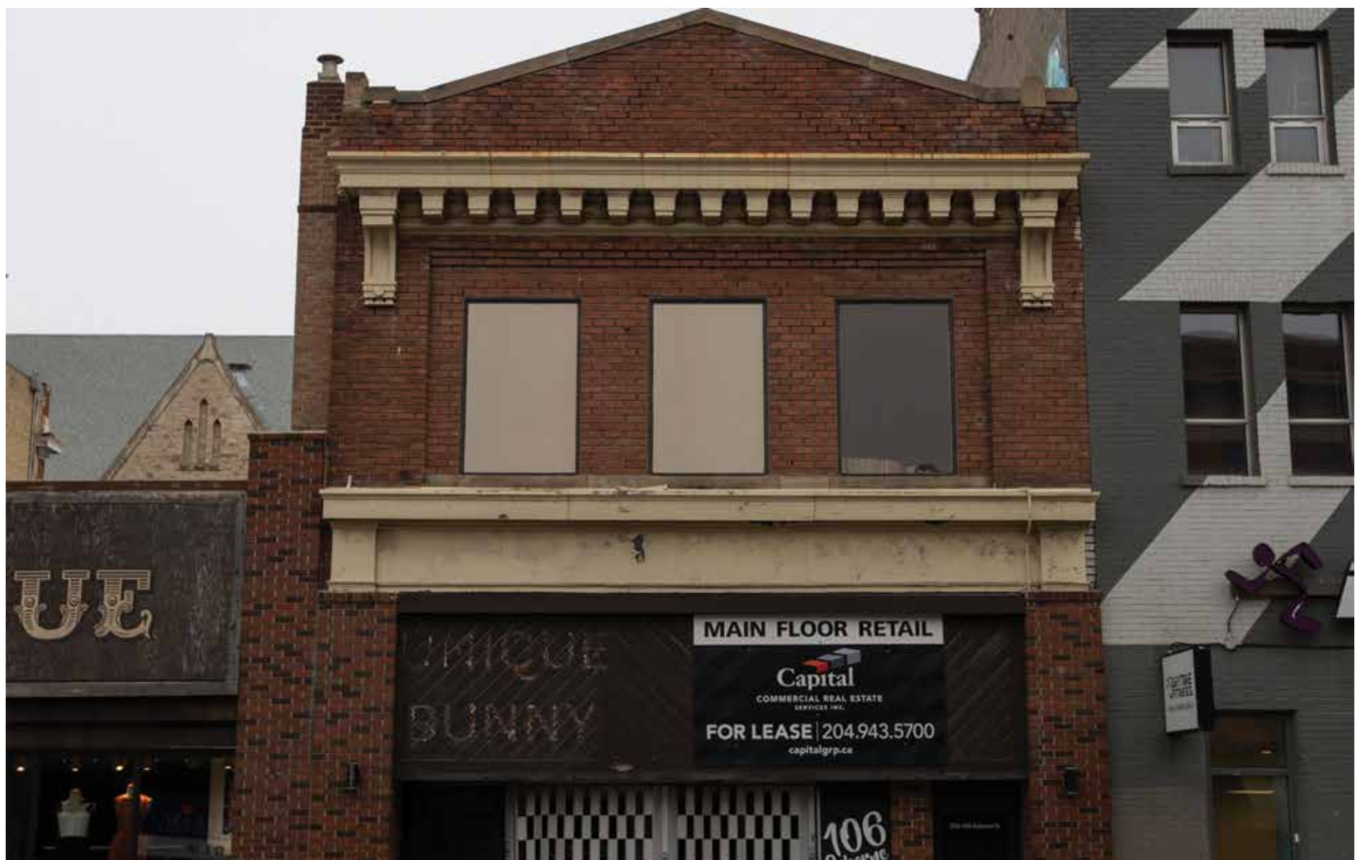
106 Osborne St., a building constructed in 1912, currently sits vacant.
