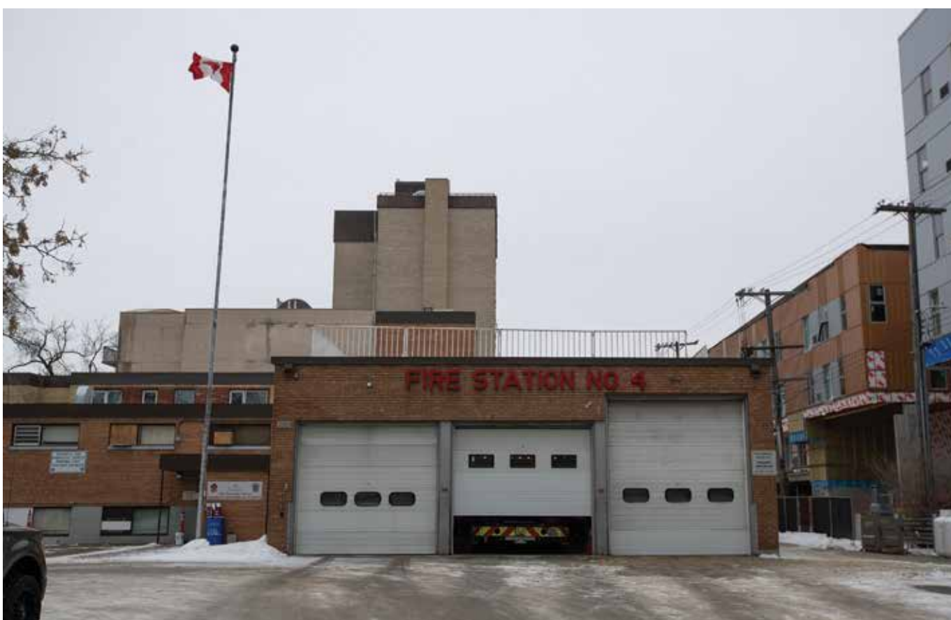
Firehall No. 4 (150 Osborne St.) was constructed in 1955.
