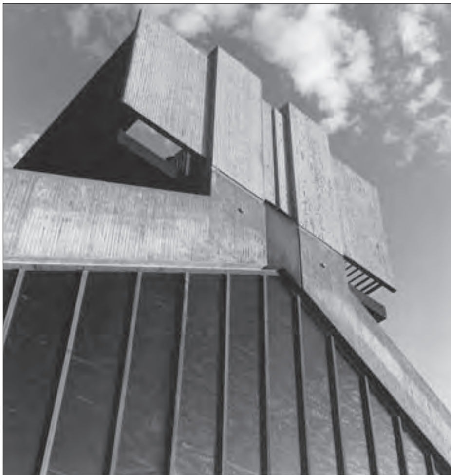
Campus Heating and Cooling Plant
